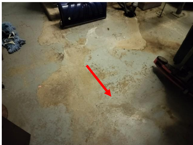
Photo 7: View of the low-level lead containing grey paint (see arrow) observed to be in fair condition on the floor within the Boiler Room.
