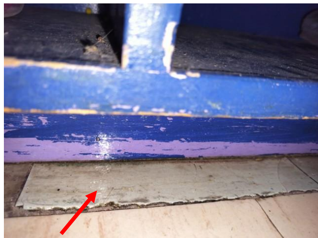
Photo 1: View of the asbestos containing 9"x9" blue/grey vinyl floor tiles (see arrow) observed to be in fair condition beneath the shelving unit within Classroom 204.
