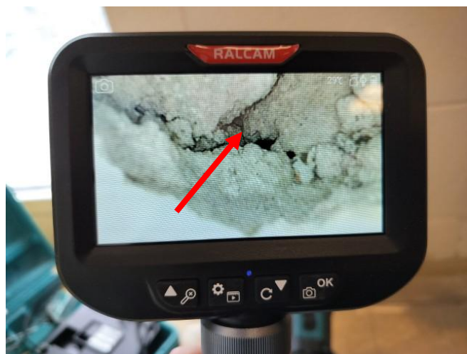
Photo 11: View of the borescope (see arrow) observing within the drill hole conducted in Classroom 210 during the vermiculite investigation.
