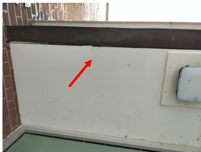
Photo 5: View of the asbestos containing cement board (see arrow) observed to be in fair condition at the exterior of Corridor 219.
