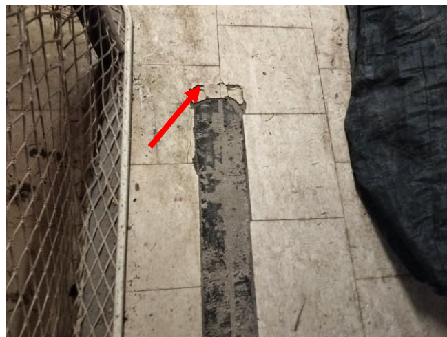
Photo 2: View of the asbestos containing 12"x12" beige vinyl floor tiles with light and dark flecks (see arrow) observed to be in fair condition within Storage Room 116A.
