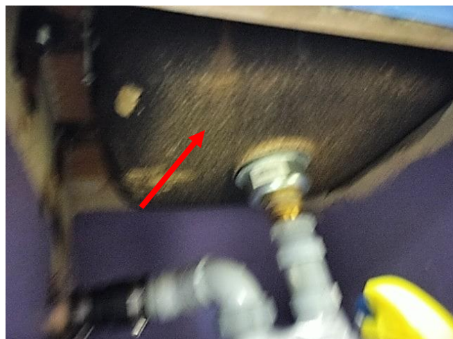
Photo 3: View of the asbestos containing gold sink coating (see arrow) observed to be in good condition within Classroom 115.
