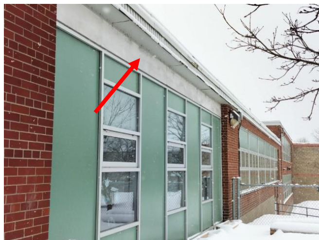
Photo 7: View of the asbestos containing cement board (see arrow) observed to be in good condition on siding near the Parking Lot of the Subject Building.
