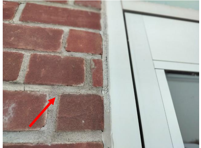
Photo 10: View of the non-asbestos containing brick mortar (see arrow) observed on the exterior walls throughout the Subject Building.
