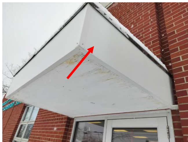
Photo 4: View of the encapsulated asbestos containing cement board (see arrow) observed to be in good condition on east exterior soffits.
