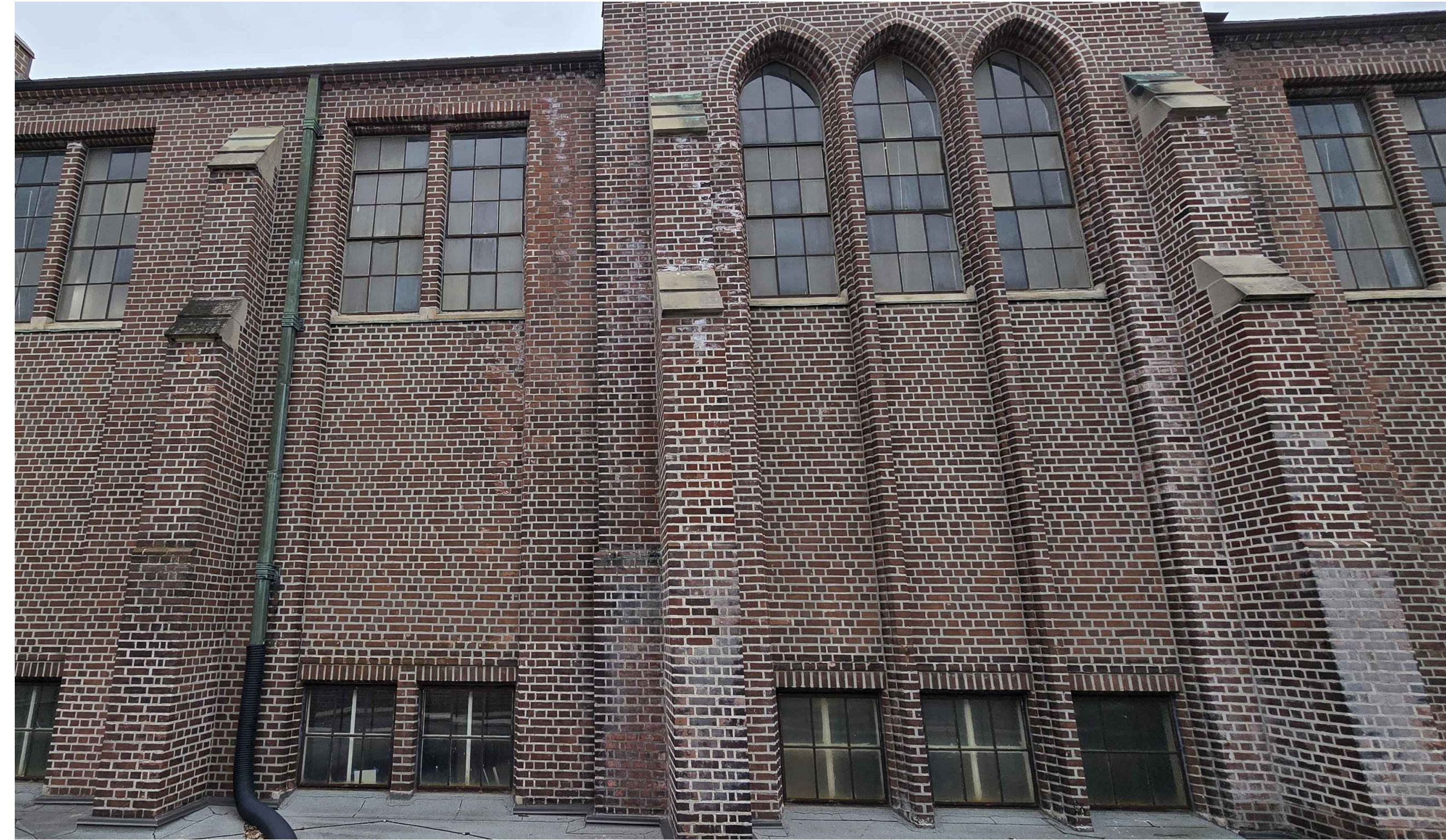
3 EX. CONDITION PHOTO 02 S301
