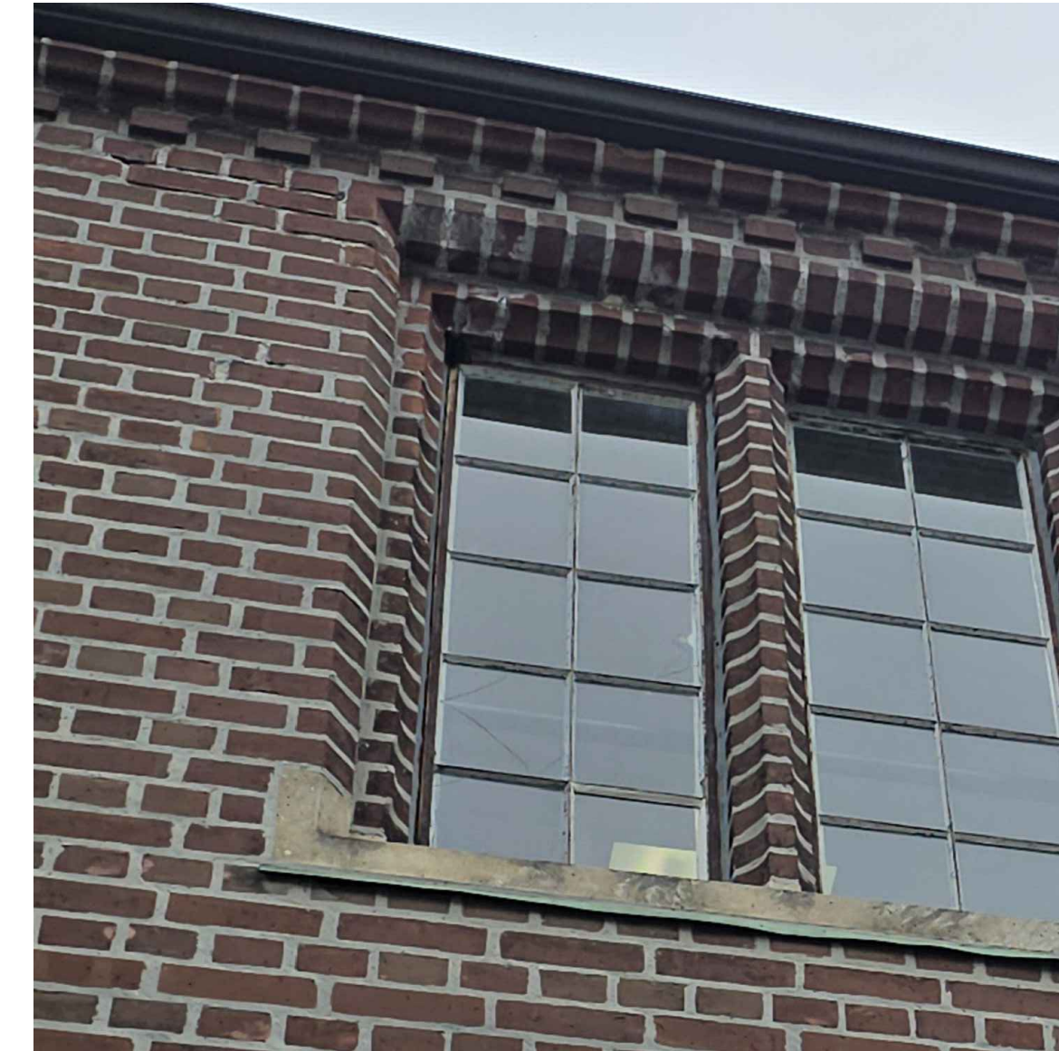
3 EX. CONDITION PHOTO 01 S302
