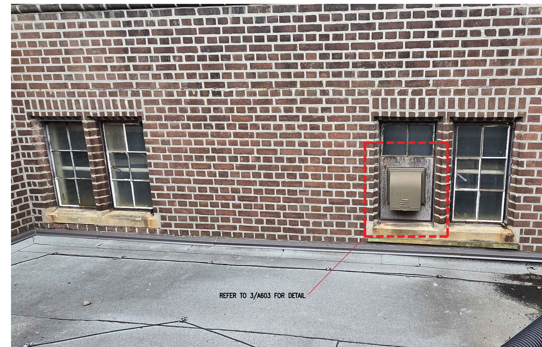
3 EX. CONDITION PHOTO 01 A602
