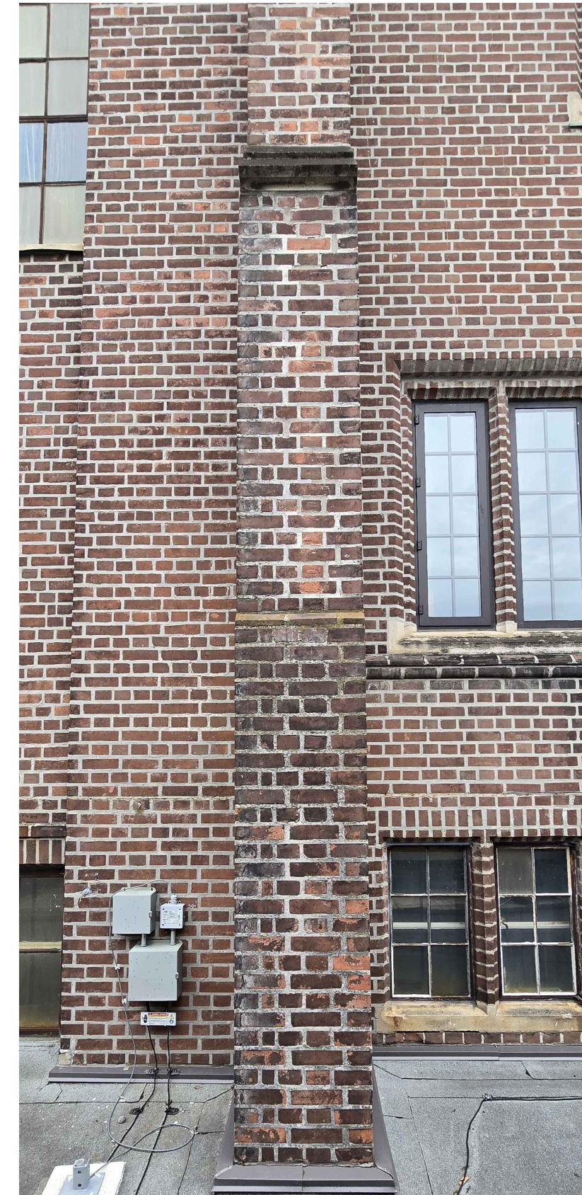
5 EX. CONDITION PHOTO 03 S302
