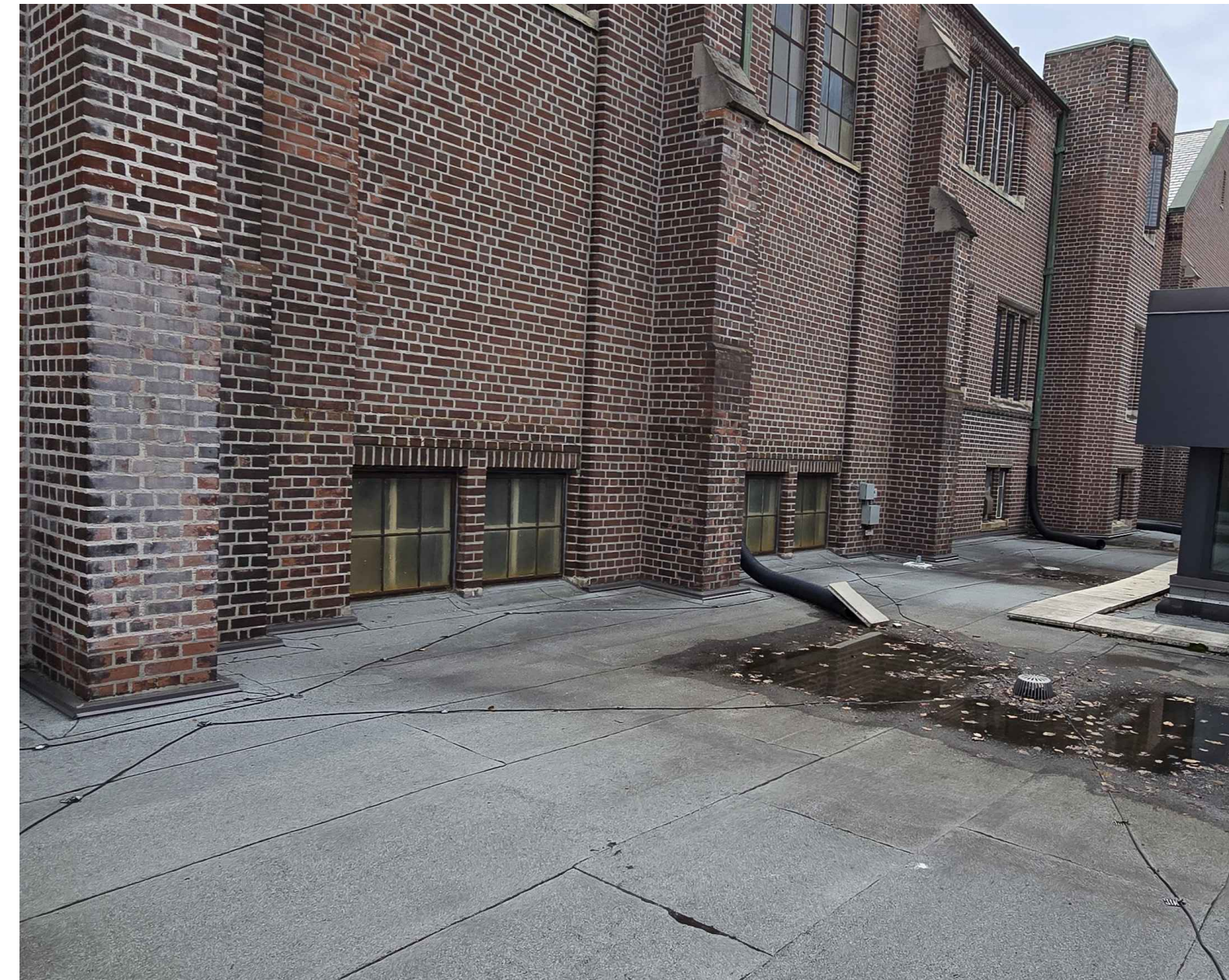
4 EX. CONDITION PHOTO 01 A201
