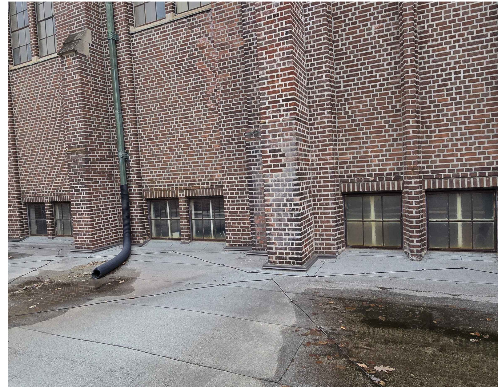
5 EX. CONDITION PHOTO 02 A201
