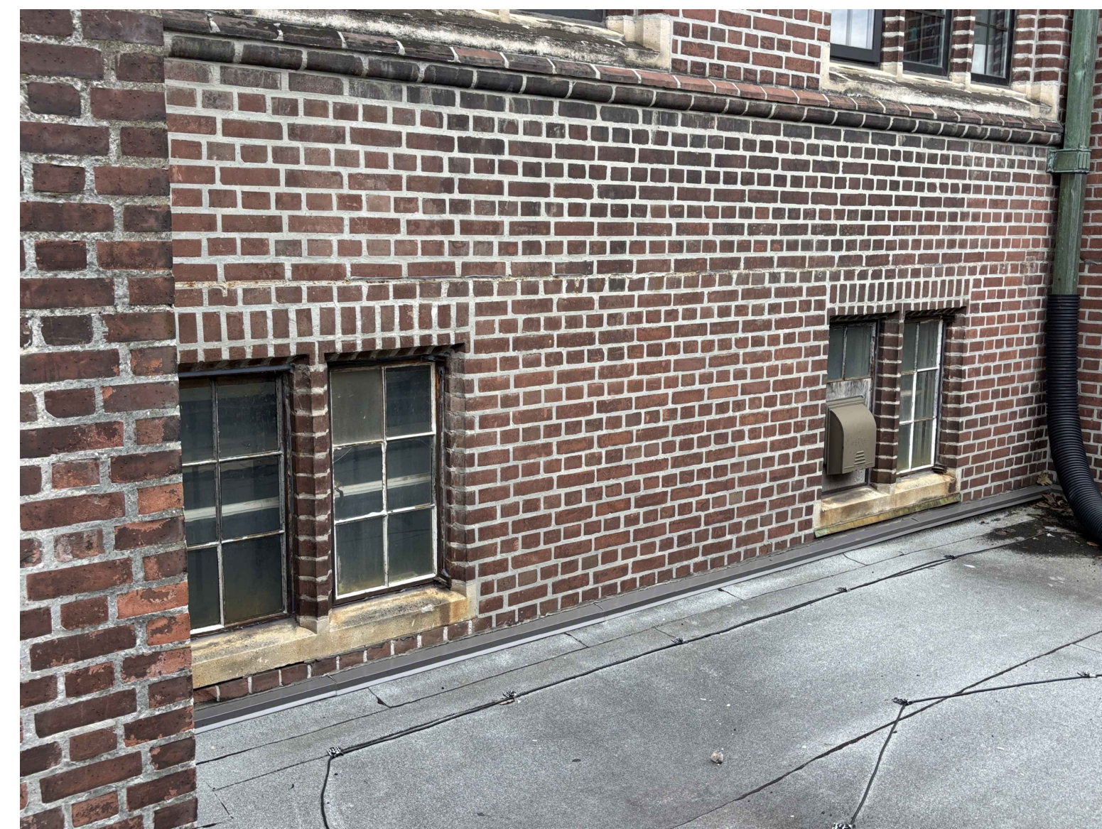
4 EX. CONDITION PHOTO 02 A602
