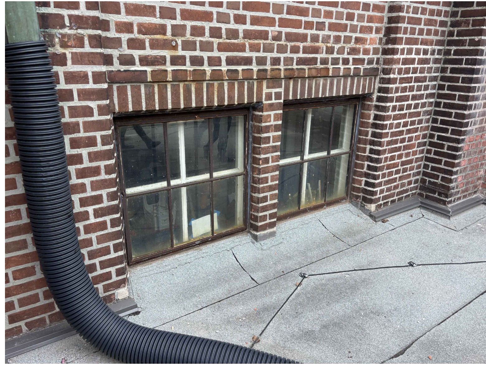
5 EX. CONDITION PHOTO 02 A601
