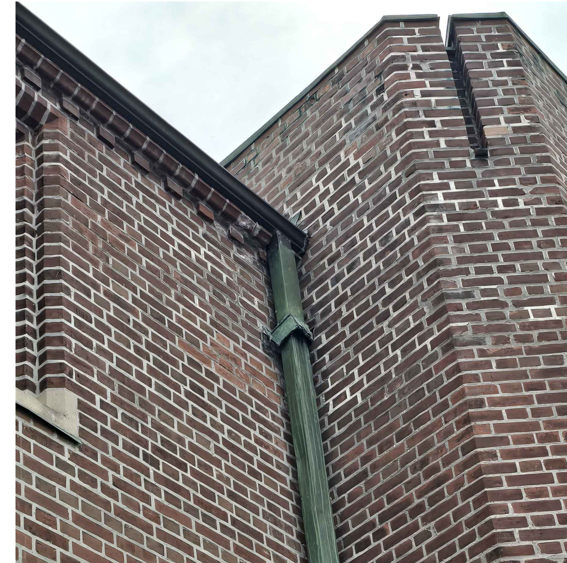
4 EX. CONDITION PHOTO 02 S302
