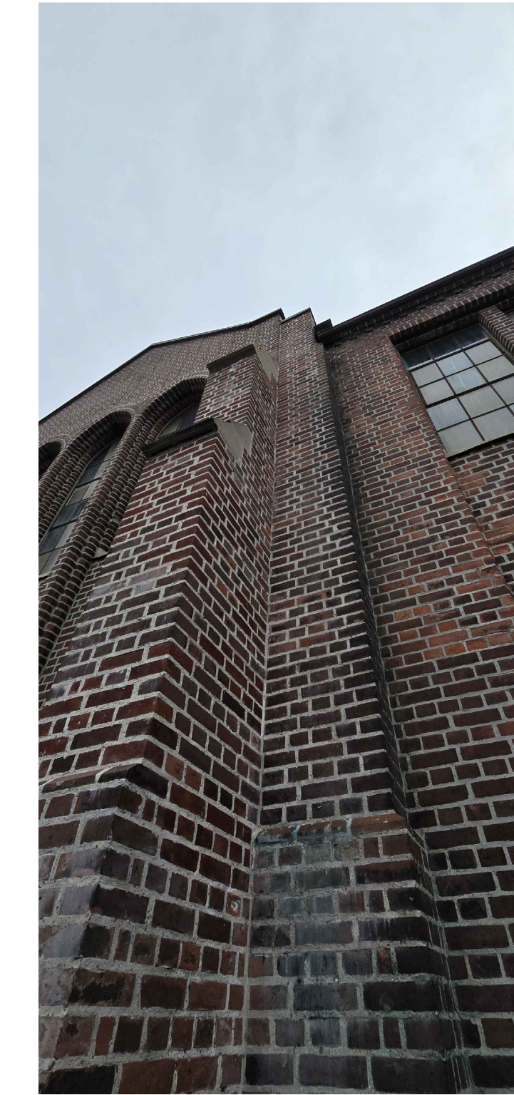
2 EX. CONDITION PHOTO 01 S301
